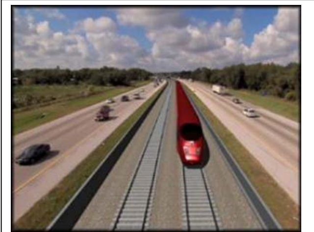
FIGURE 3: The computer rendering above depicts a typical condition within Interstate 4 where the HSR alignment would be contained in the center median. (SOURCE: www.wtsp.com , Tampa Bay Ch. 10 News)
